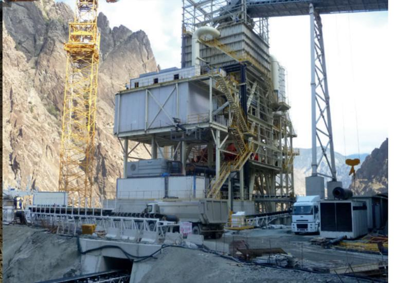
Aggregate is one of the biggest components in the concrete mix and hence its effect on concrete temperature is very high. By lowering the aggregate temperature by approx. 2°C, fresh concrete temperature will drop by 1°C.
