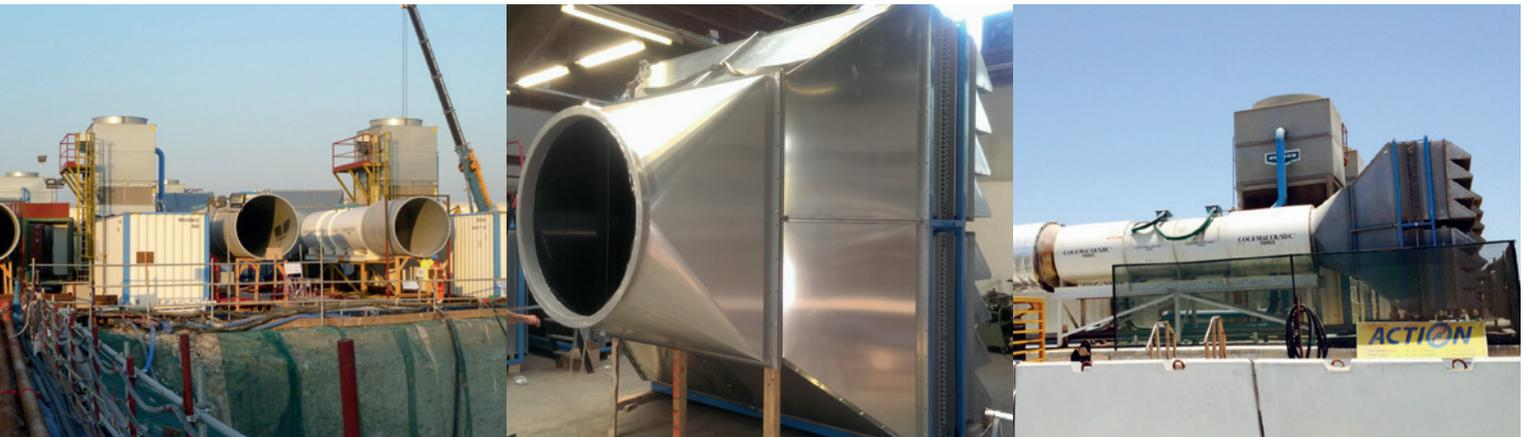
There are strict rules about the working climate inside tunnels and mines. Ventilation requirements are dictated by the desired conditions.
