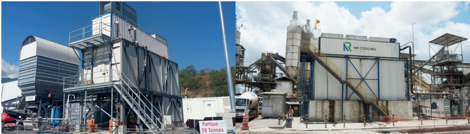
The most frequently applied cooling method for lower fresh concrete temperatures is replacing the mixing water by flake ice.
